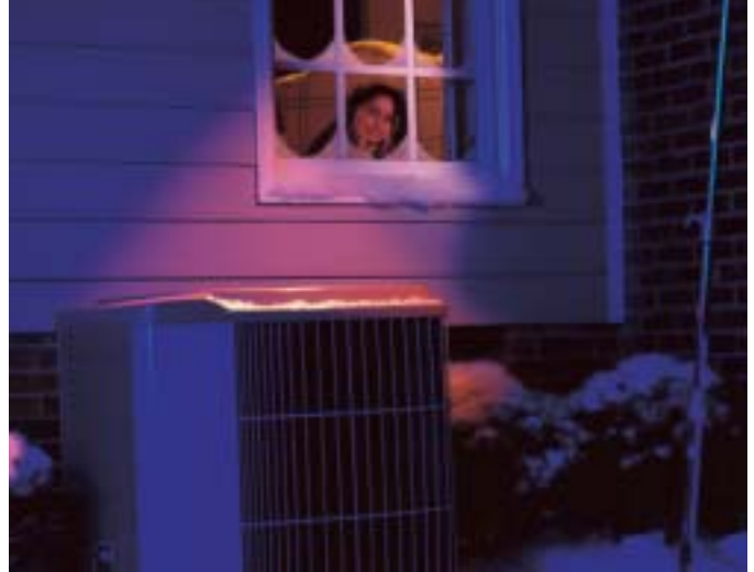
During mildly cold weather, the heat pump is less expensive to operate than the furnace. As the outdoor temperature drops and the heat pump becomes less efficient, the gas or oil furnace takes over.
